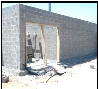
Traylor Stadium Renovations
