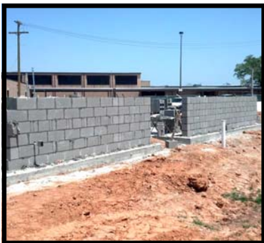
Traylor Stadium Renovations
