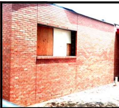
Miscellaneous Renovations / Jackson ES
