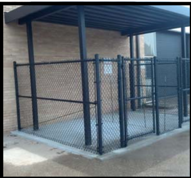
Miscellaneous Renovations / Lamar HS
