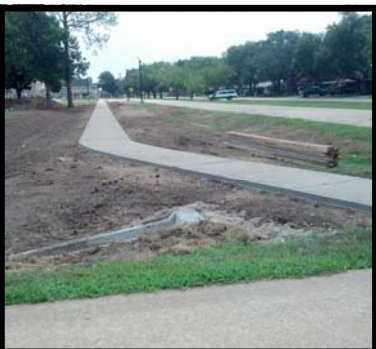
Miscellaneous Renovations / Bowie ES
